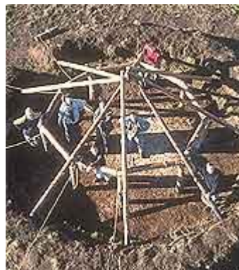
Howick house - under construction ©
