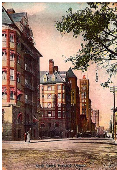
This image of Sixth Street in downtown Portland
