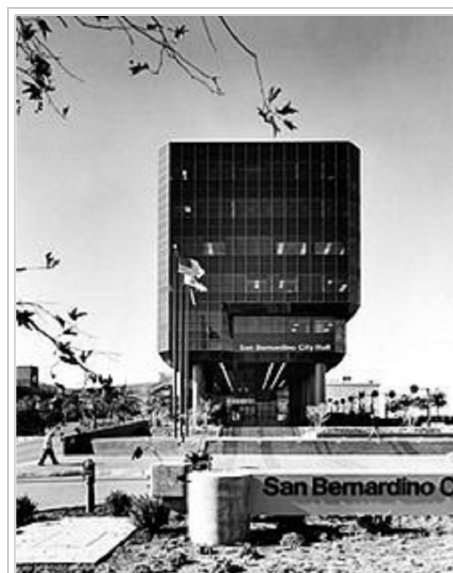
San Bernardino City Hall building designed by César Pelli.
